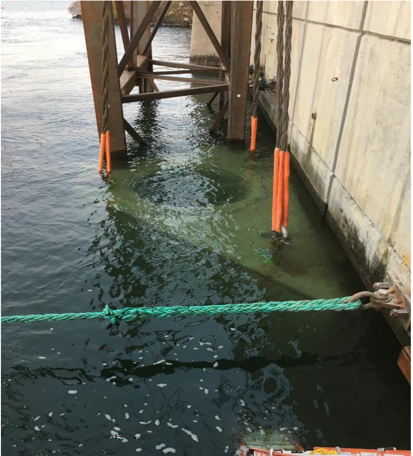
Peirnose block installation underway in forebay.
